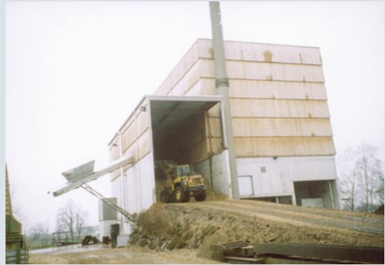
Above: A vehicle loading wood waste into the Biostrom plant
