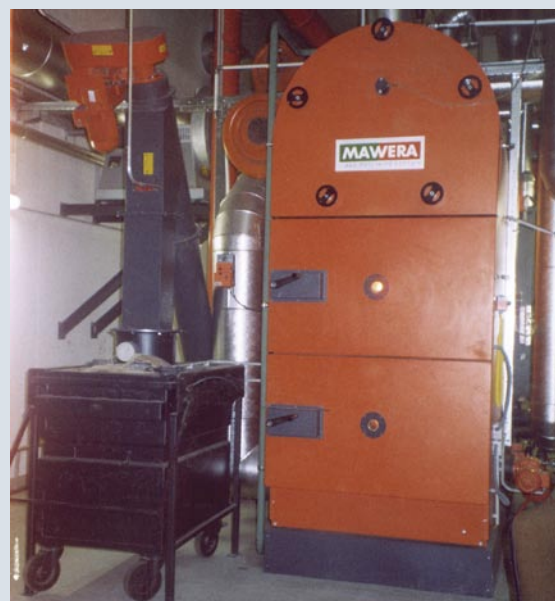
The picture on the left shows the other end of the boiler. The Stirling engine is contained within the orange box mounted half-way up the boiler.
